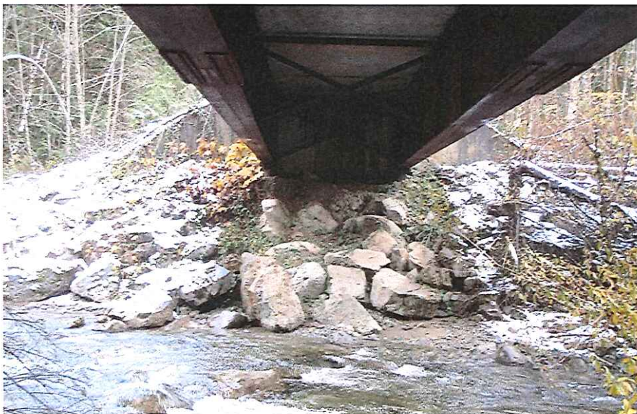
CK-2042 Abutment Right Bank
