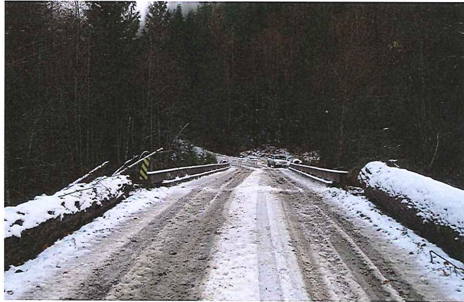
CK-2042 Approach Right Bank
