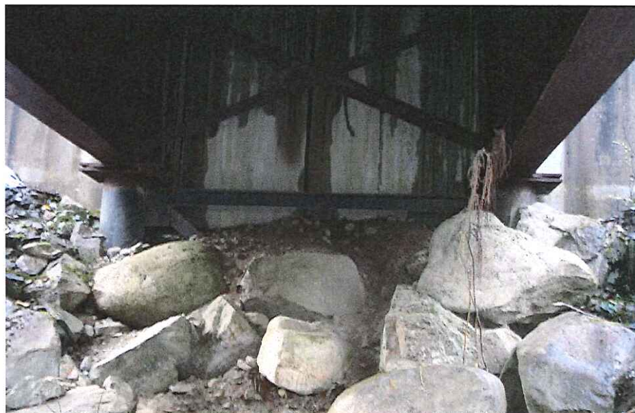
CK-2042 Abutment Left Bank #2
