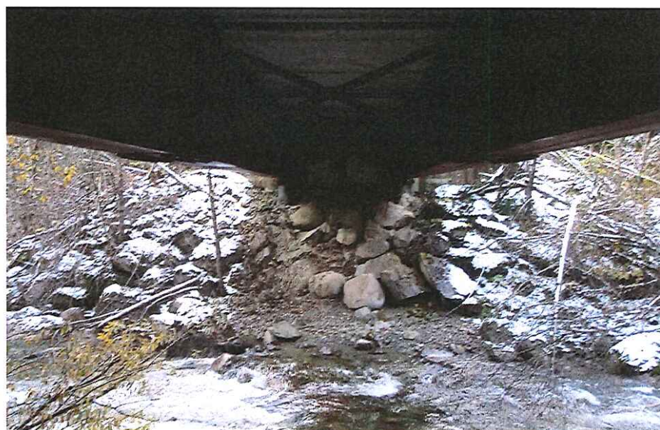
CK-2042 Abutment Left Bank
